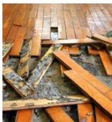
Leak Under The Floor
