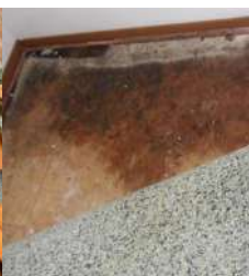
Leak Under The Floor
