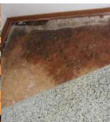
Leak Under The Floor
