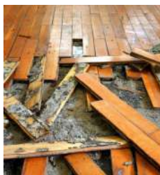
Leak Under The Floor
